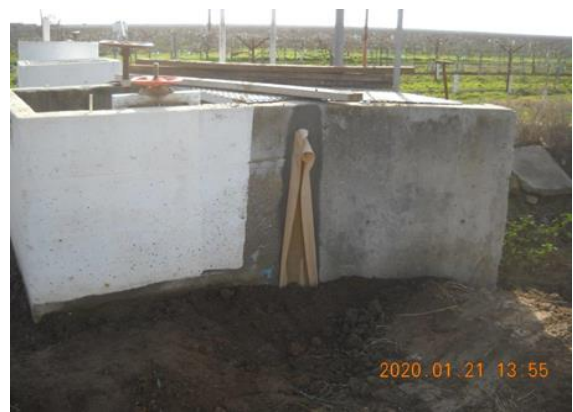
Colony Ext. Pipeline structure leak repaired
