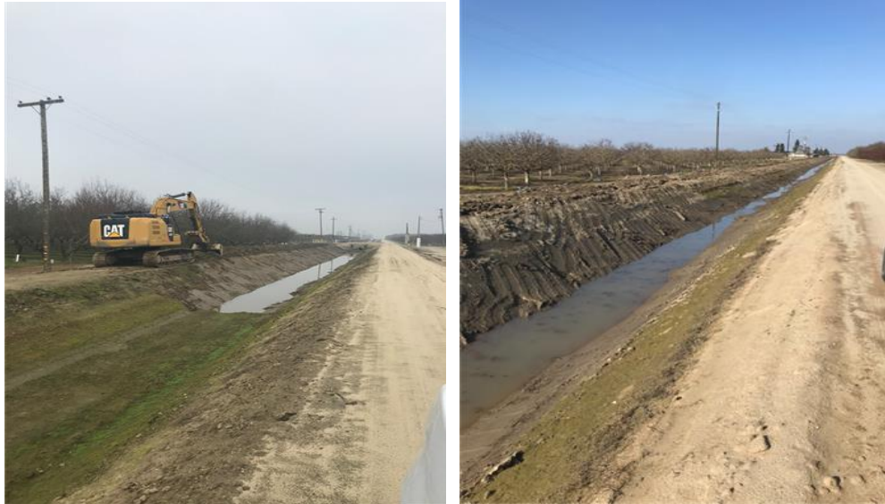
Canal dredging on 24.2 north of Ave. 12 and south of Ave. 13 ½
