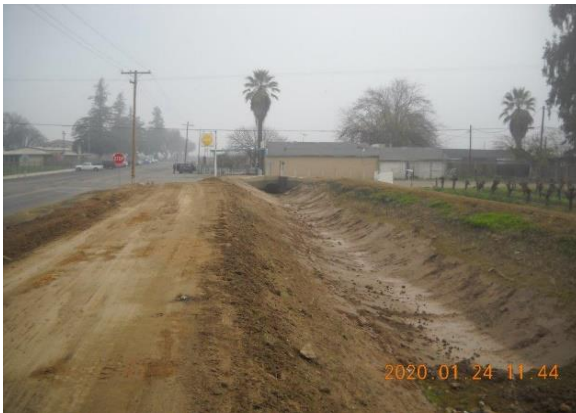
Grading on the 15.9 at Ave. 8 and Rd. 30
