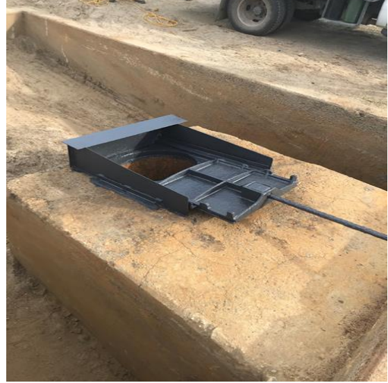
Madera Lake Dam slide gate repaired
