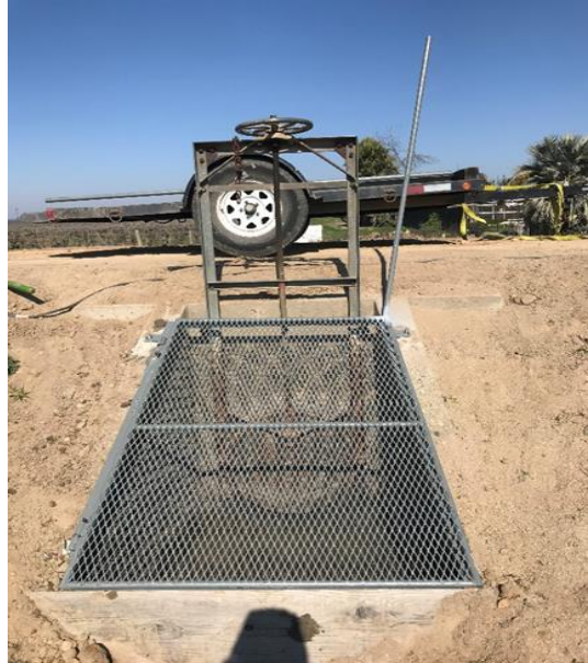
Trash guard on the 6.2 Ext & head on 21.1 Trash screen on the 15.9 turnout #7
