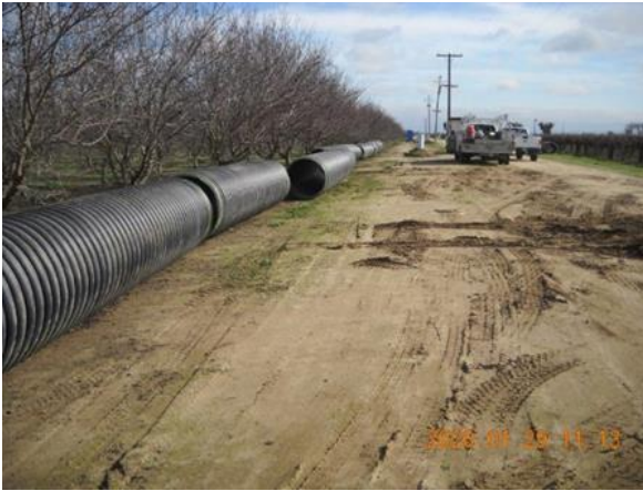
Replacing 2,600 ft. of cracked concrete pipe with new 36” ADS Pipe on the Colony Ext. located between Rd. 20 and Rd. 20 ½.
