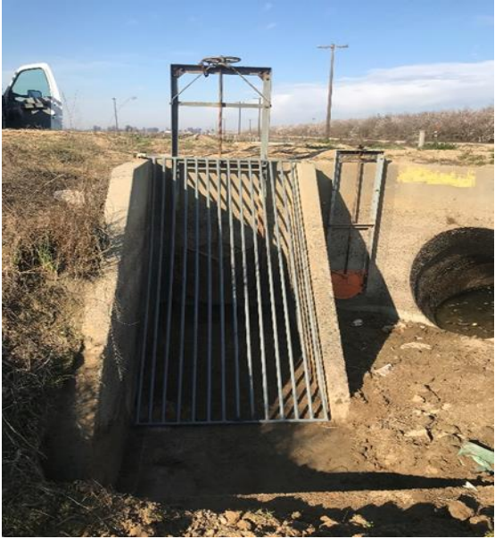
Trash guard on the 6.2 Ext & head on 21.1 Trash screen on the 15.9 turnout #7
