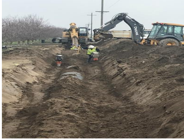
Replacing 2,600 ft. of cracked concrete pipe with new 36” ADS Pipe on the Colony Ext. located between Rd. 20 and Rd. 20 ½.
