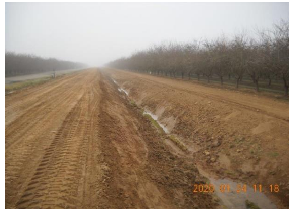
Canal grading and sloping on the 6.2-15.9
