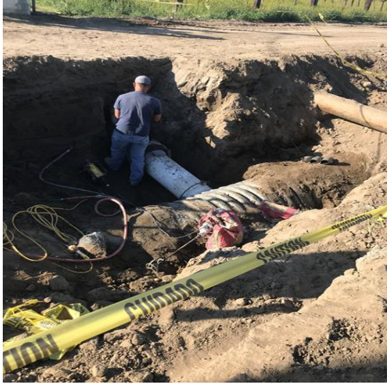
Colony Ext. pipeline turnout tie in
