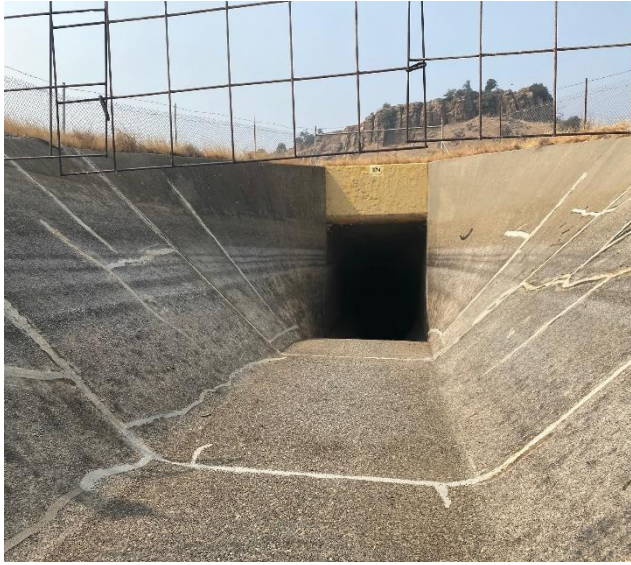
Sikaflex The Downstream Side of Siphon #3
