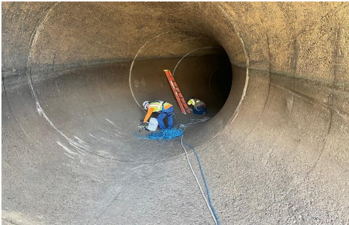
Sikaflex Sealant Applied Siphon Joints
