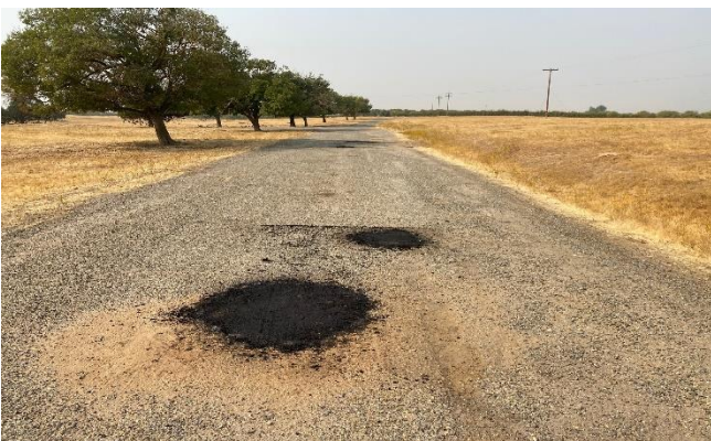
Madera Lake Entrance Road Repaired
