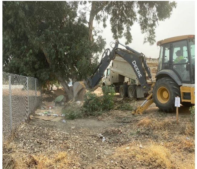
Clean-up Along the 24.2 Canal
