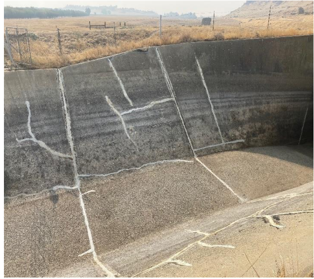
Sikaflex The Downstream Side of Siphon #3
