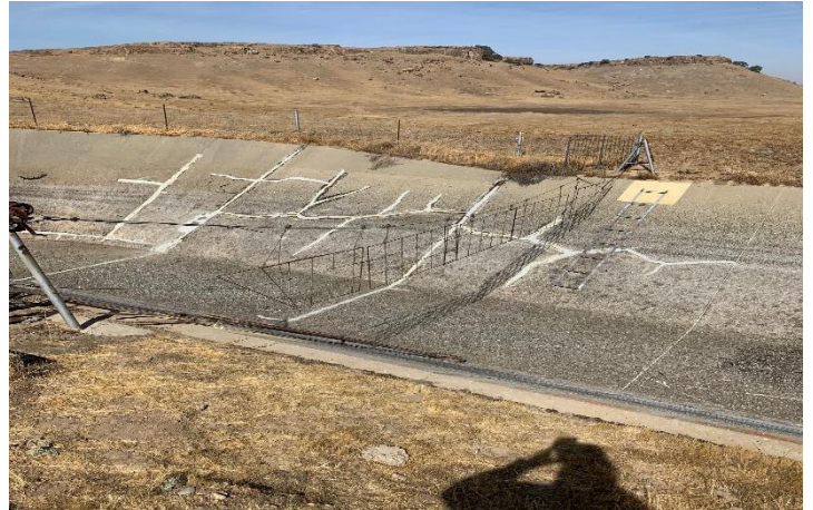
Sikaflex Applied Concrete Panels
