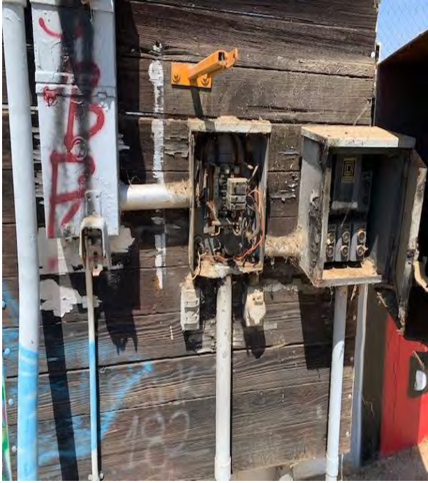
Basin #8 Road Crossing
