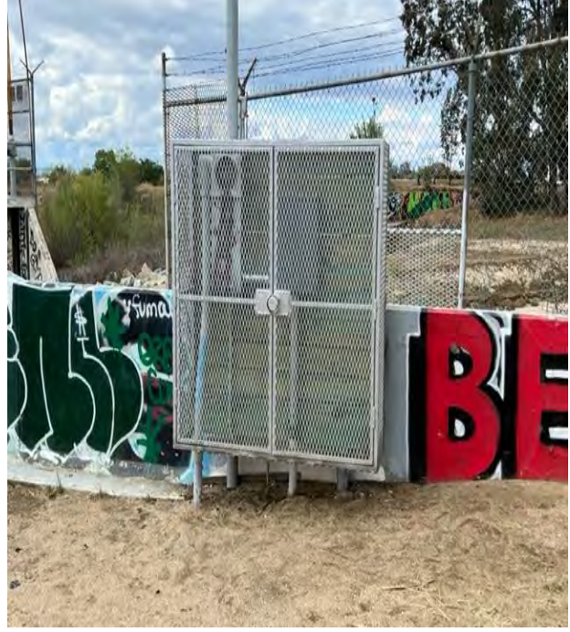
Clark Pipeline Repairs
