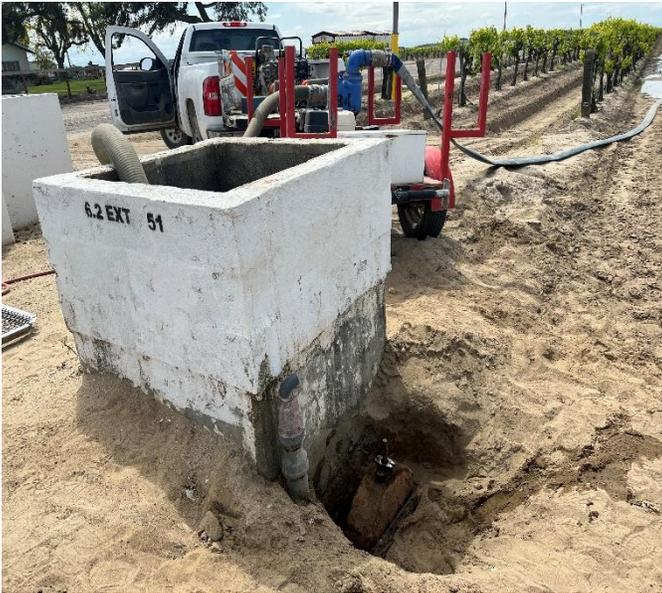
6.2-16.9 Installed New 15 Inch Gate Valve
