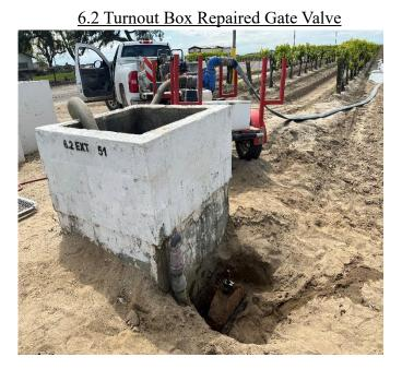
6.2-16.9 Installed New 15 Inch Gate Valve
