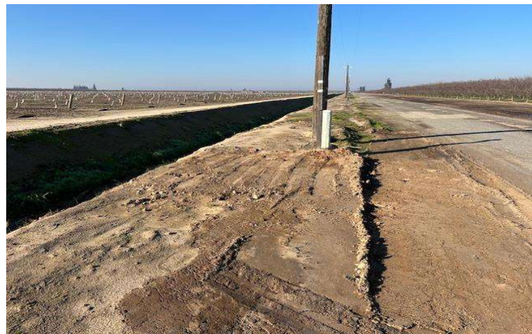
Colony Extension along Avenue 13.5 – Repaired Washout
