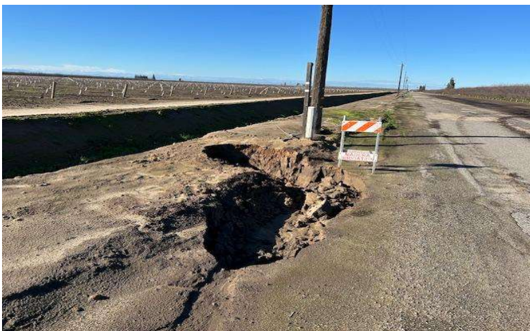
Colony Extension along Avenue 13.5 – Repaired Washout
