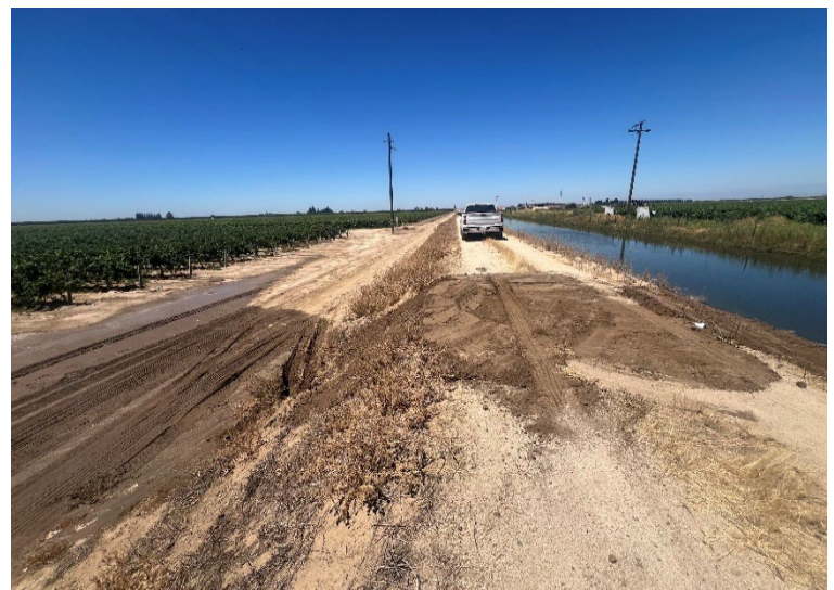
24.2 North of Avenue 14 – Repaired Gopher Hole on Canal Bank
