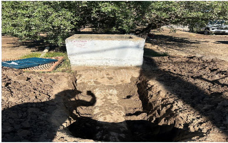
Repaired Turnout Box – Schmitz
