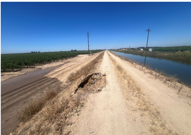
24.2 North of Avenue 14 – Repaired Gopher Hole on Canal Bank
